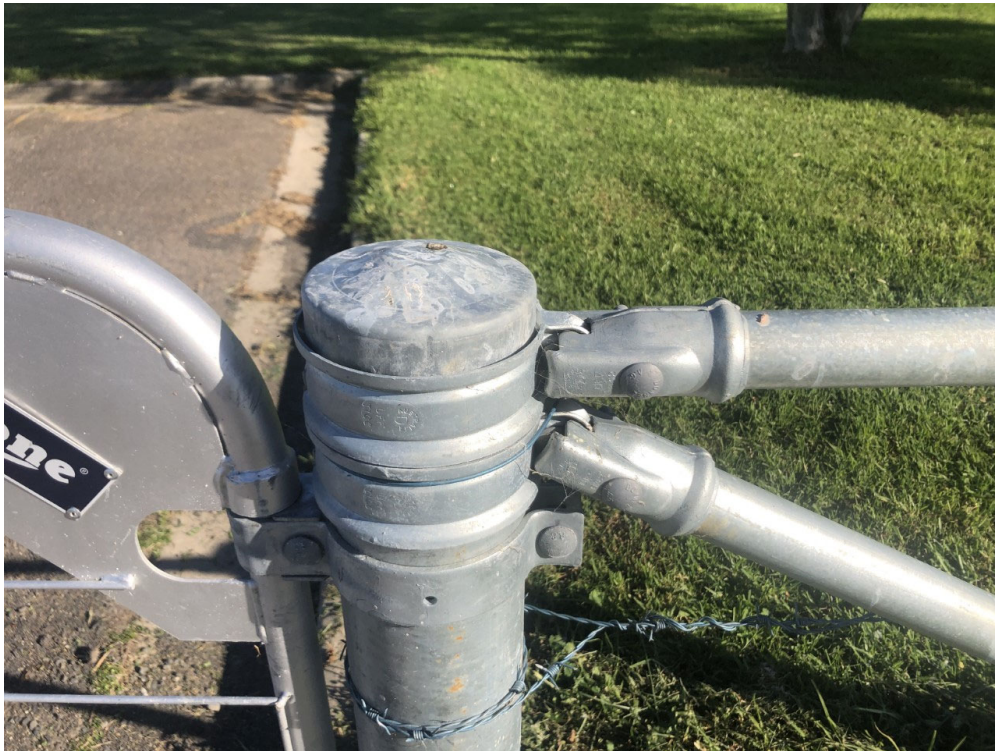
Detail showing stay and gate post connection
