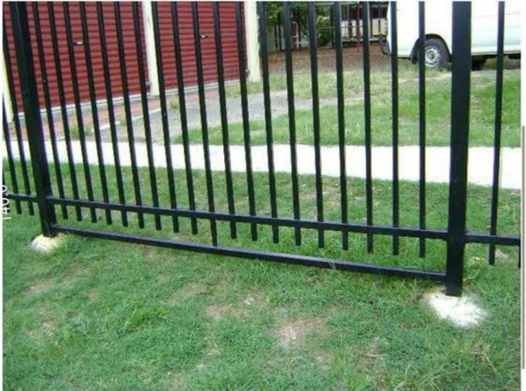
Bottom Infill Rail Detail
