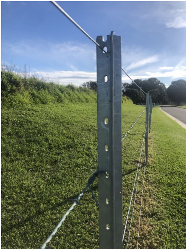
Star picket and wire runs for internal fencing
