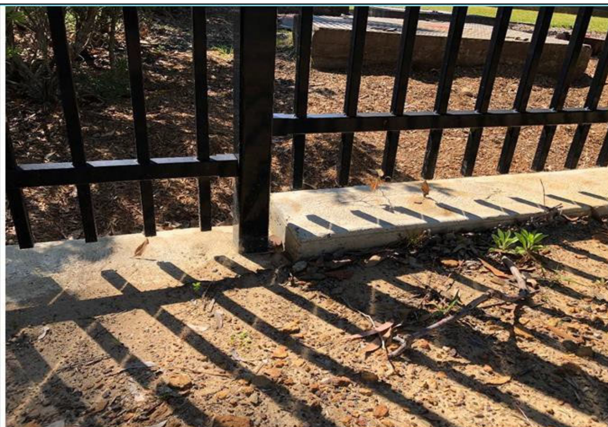
Details Showing Stepping of Concrete Kerbing
