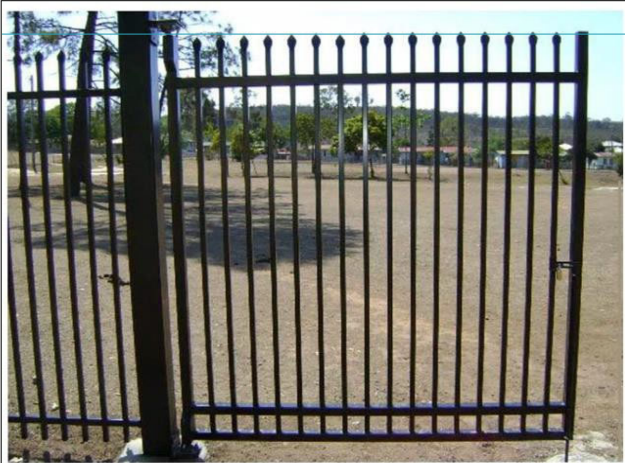
Gate Detail showing twin bottom rails
