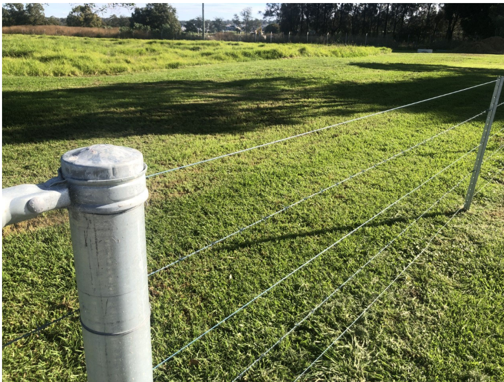
Galvanised barbed wire runs with star picket
