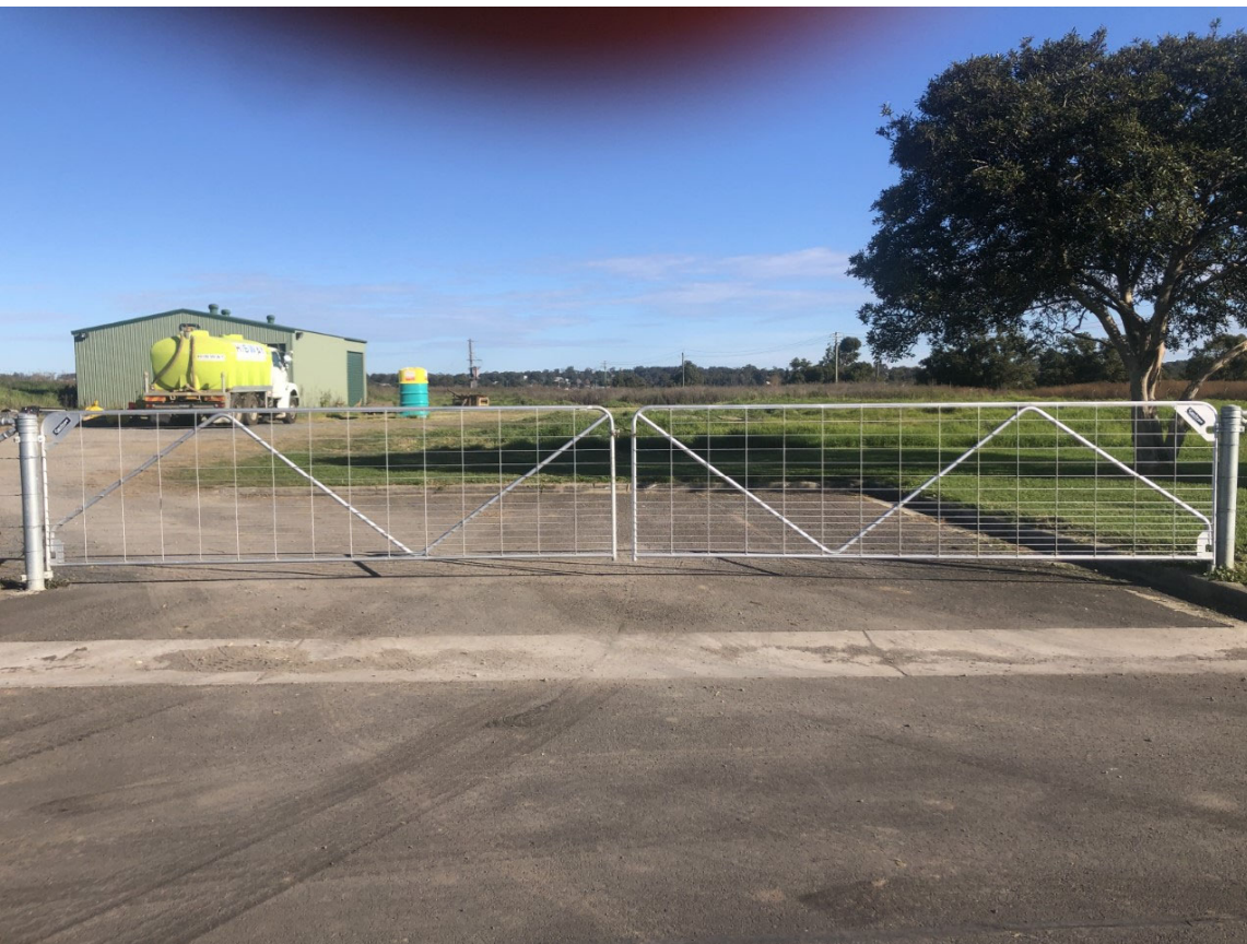
Double 4.2 m galvanised stock gate
