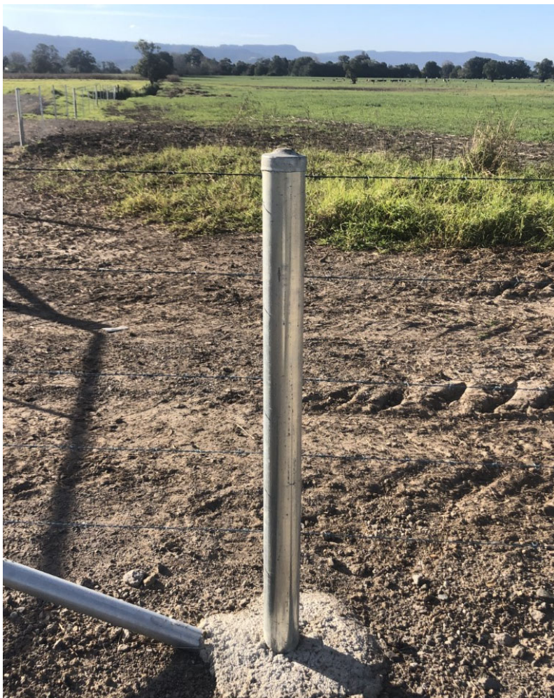
Detail showing intermediate post for boundary fencing
