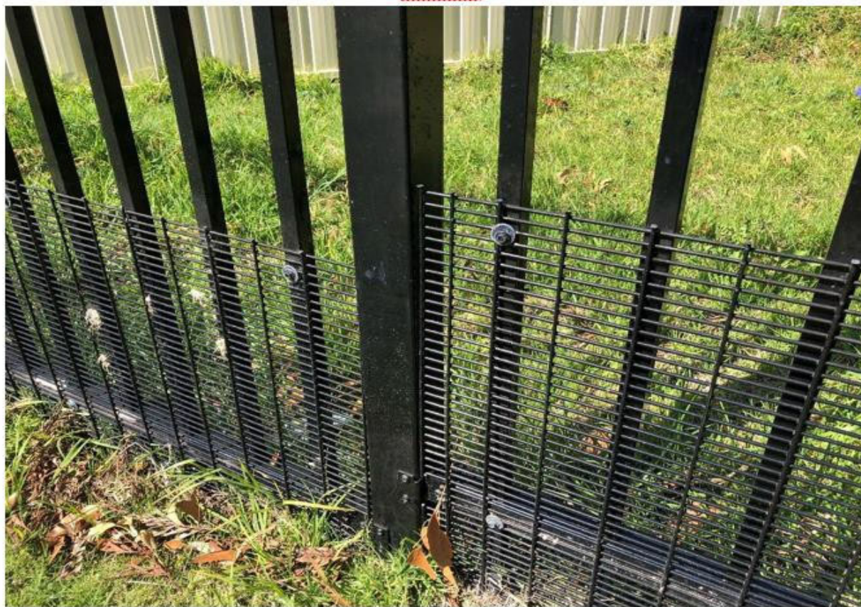
Animal Barrier Mesh Detail
