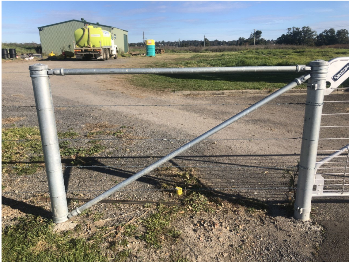
Detail showing gate post and stay
