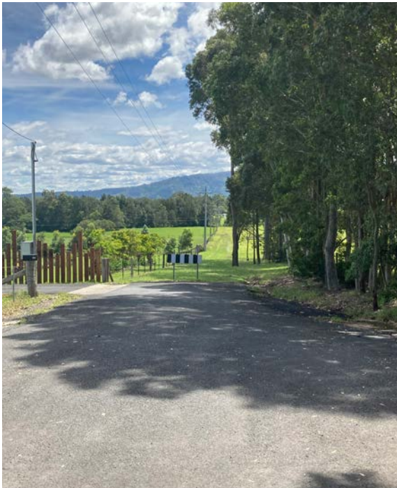
◀ Termination of sealed road providing driveway access to Taylors Lane properties.
