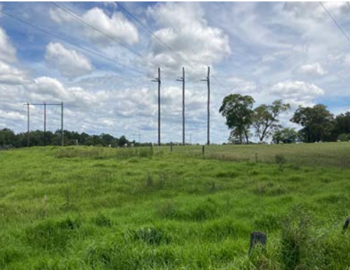
Overhead power lines crossing Taylors Lane
