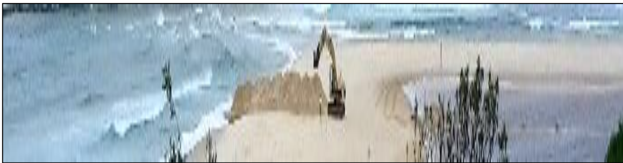
Figure 4-1 Excavation of the Pilot Channel on 17 March 2017
