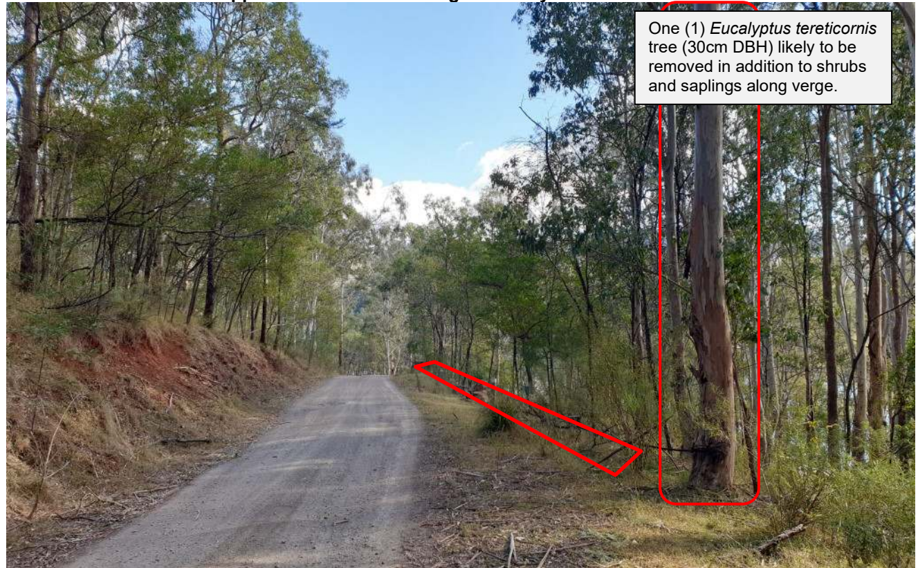
Photo 6. Access road at approx. Ch. 400 m showing tree likely to be removed
