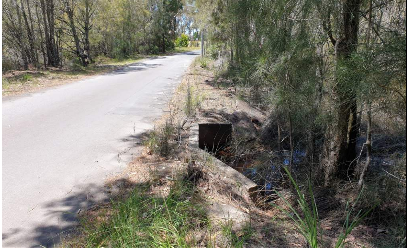
Photo 4. Berry St culvert crossing showing one of the two twin-pipe-culverts
