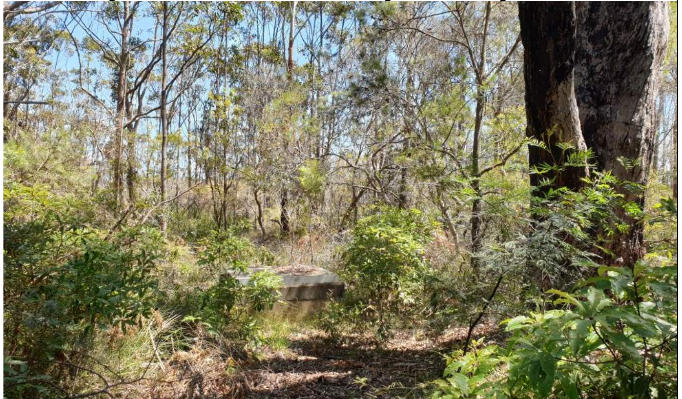
Photo 12. Existing manhole to the west of SPS7 where existing overflow discharge occurs.
