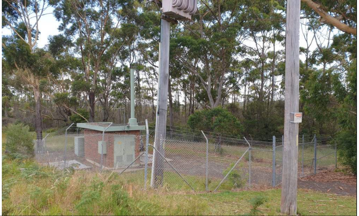
Photo 11. Existing sewer pump station SPS7 compound
