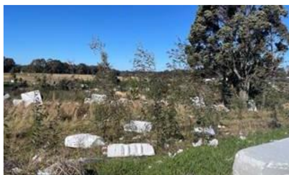
Badagarang – Pollution incident Polystyrene pods blown from a building site
